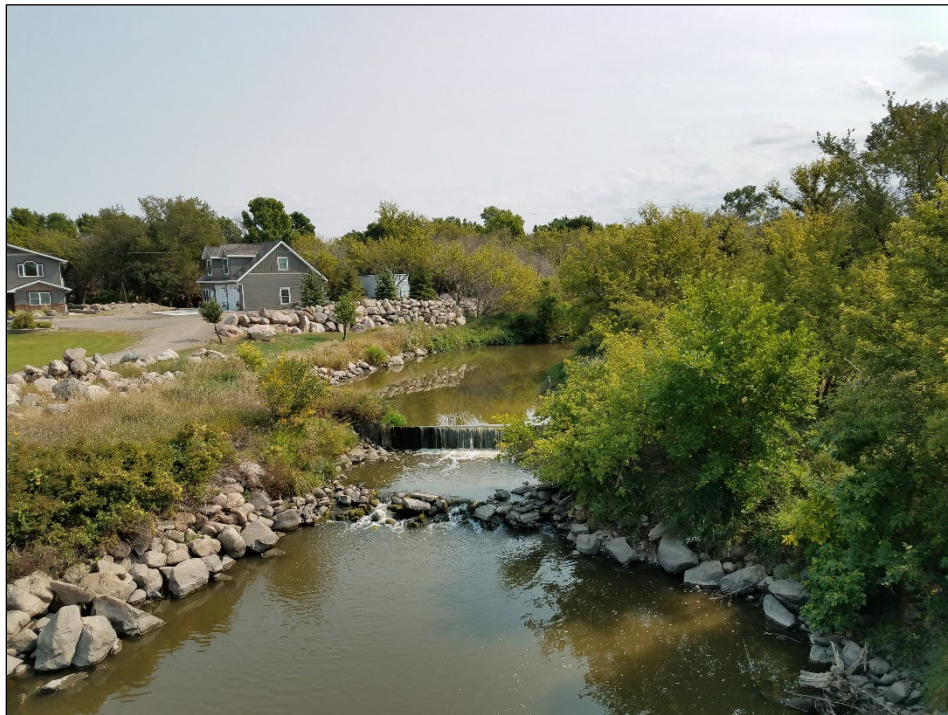
Beaver Creek low-head dam west of the City of Linton.
