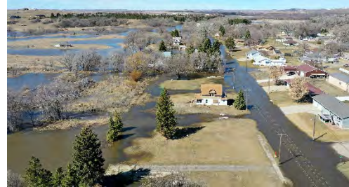
Sampson Avenue looking West.
